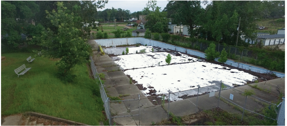
The current state of Ruston Memorial Park City Pool.
